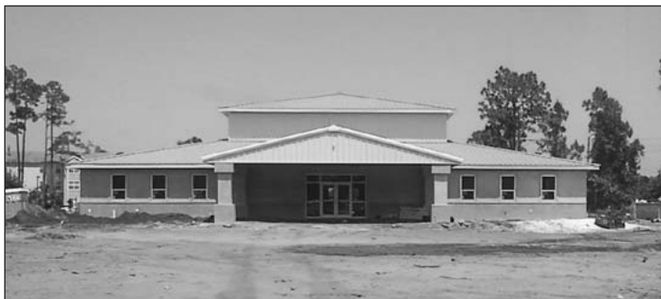
Current building as it is today.
